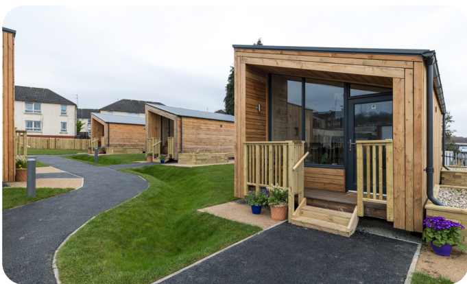
Houses at Social Bite Villages are delivered to an exceptional standard in order to provide a beautiful, dignified and high quality home for residents
